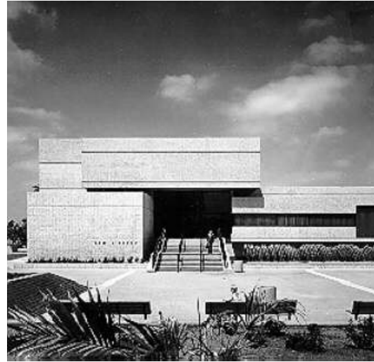
Image Source: Orange County Public Law Library http://www.ocpll.org/FACILIT.HTM
